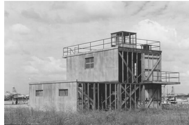
Back, Base Operations/ Control Tower
