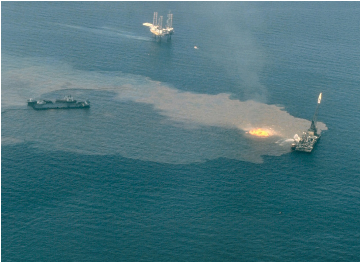
Figure 4. Ixtoc I exploratory oil well burning in water at 160 feet depth poured 380 million gallons of crude oil from 3 June 1979 to 23 March 1980 after a 10 month effort to seal the well.
